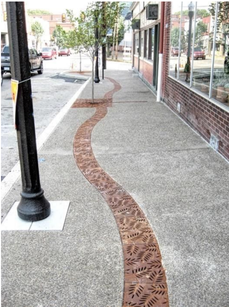
Storm water management in Etna doubles as attractive street art. Permeable sidewalks and decorative drains direct water and prevent flooding.
