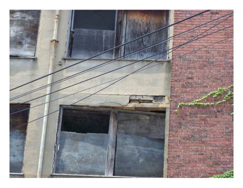
Photo 8 – Open Window / Façade Deterioration
