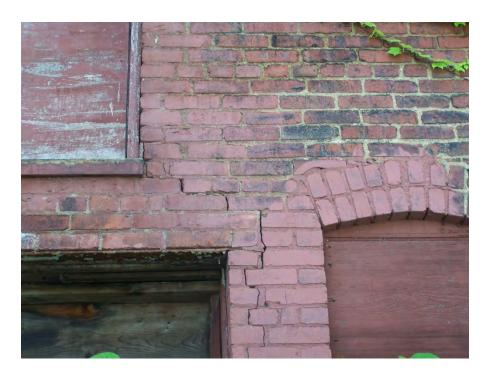
Photo 5 - Cracked Brick (due to corroded lintel)
