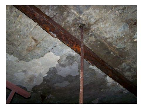
Photo 2 - Corroded Steel Beam - No Concrete Cover
