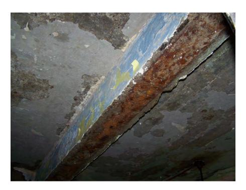
Photo 3 - Corroded Steel Beam (some concrete cover)
