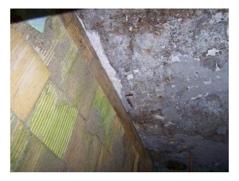
Photo 4 – Spalling of Bottom of Concrete Floor
