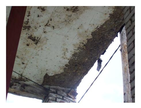
Photo 7 – Concrete Deck Deterioration
