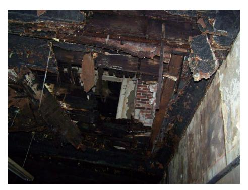
Photo 3 - Deteriorated Wood Floor Structure
