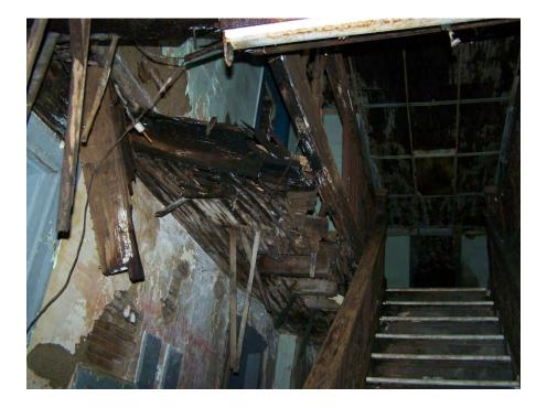
Photo 2 - Deteriorated Wood Floor Structure
