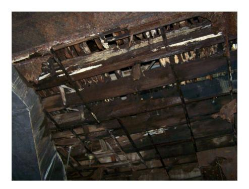
Photo 1 – Deteriorated Wood Floor Structure
